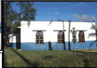
Masjid at Kaliangombe, near Taqwa Centre completed in Nov 2010.
