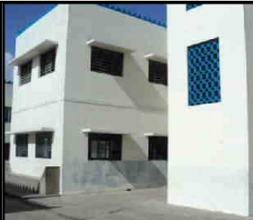
Darul Ulum Madrassa Renovation works in progress—Dec' 10
