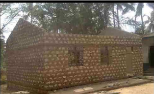
Construction of a Community Classroom project at Kwa Randu in progress
